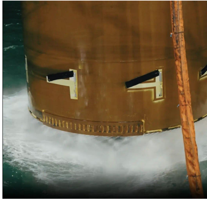
Figure 1: Lower-noise-technology used to install monopile foundations at Gode Wind 3 in Germany [8].
