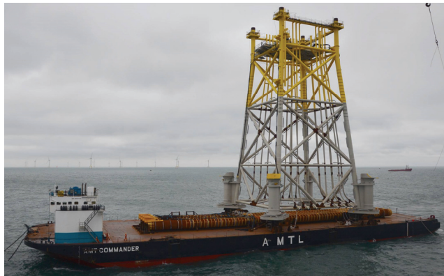
Fig.1: Typical example of a skirt pile jacket before installation, with the skirt sleeves visible at the lower end of the jacket legs.
