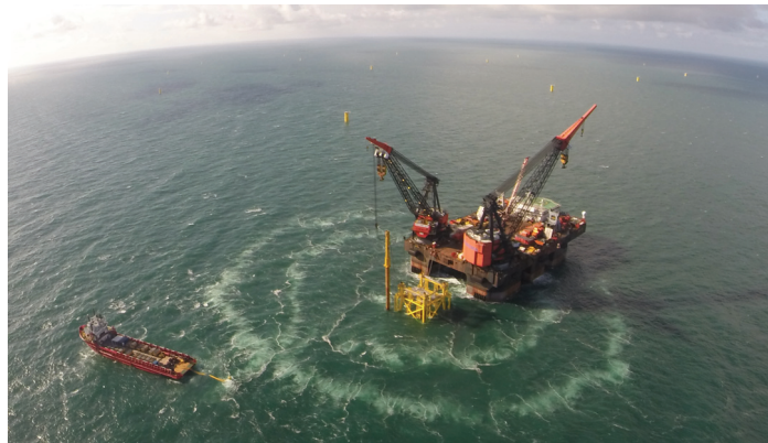
Fig.2: Situation during pile driving: hydraulic hammer visible on top of a skirt pile, with the double big bubble curtain (DBBC) active.
